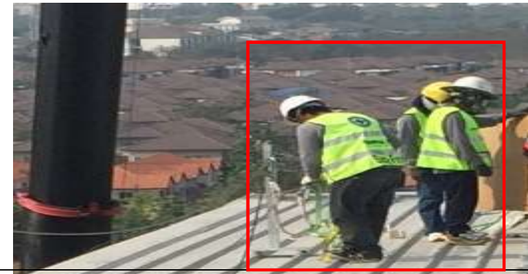
Worker did not use safety belt while working on the roof (10 m.)
